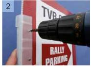
Secure the signAclip to the flute board by inserting 2 x 6 gauge screws into the clip.
