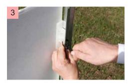
Re fit the sign to the 1<sup>st</sup> star picket & position the upper signAclip over the 2<sup>nd</sup> predrilled hole. Secure the clip to the picket with a cable tie. Also secure the lower signAclip to the 1<sup>st</sup> star picket.
