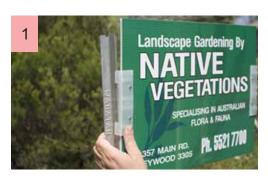
Correctly fit the sign/clips to the 1<sup>st</sup> star picket and rotate the picket until the correct sign direction is achieved. This obtains the correct fin direction for the 1<sup>st</sup> star picket.
