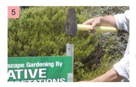
Holding the signAclips onto the picket, hammer the 2<sup>nd</sup> star picket into the ground, letting the clips slide along the star picket. Hammer the 2<sup>nd</sup> star picket to the same height as the 1<sup>st</sup>.
